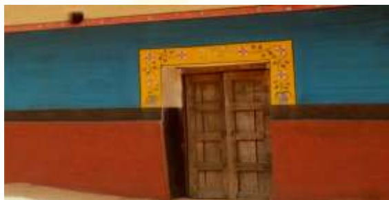
Figure 7: Decorative door and window
