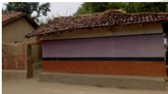
Figure 4: Horizontal division of wall
